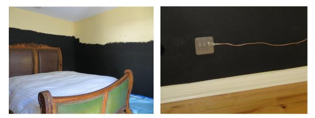
It is imperative that all E-field shielding surfaces are connected to a proper grounding system and continuity of conductance of shielding surfaces is achieved. Any grounding work should be conducted by a licensed and experience electrical contractor. Grounding is also important part of electrical safety in such a project. After two walls are now shielded, the measurements are repeated. The graphic below shows the results obtained afterwards.
